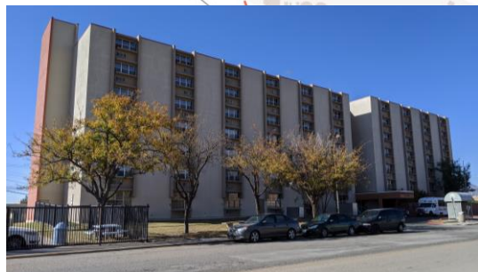
Existing Conditions at Cortez Plaza, 201 Cortez Dr.
