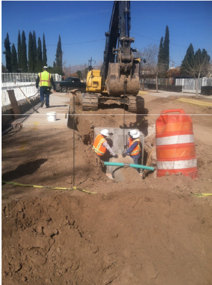
Installation of a new Storm Sewer Drainage System
