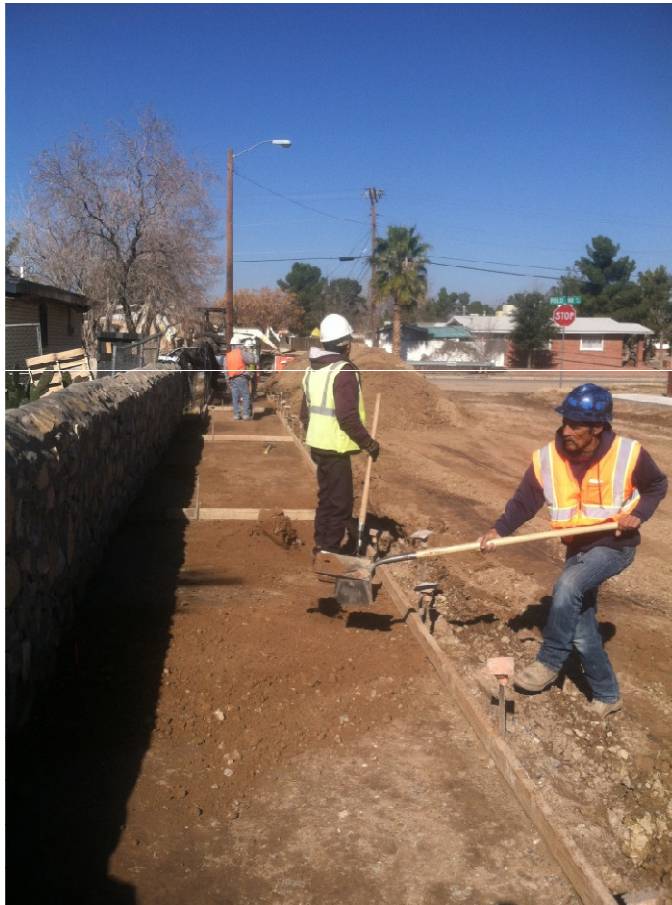
New Concrete Sidewalk Installation
