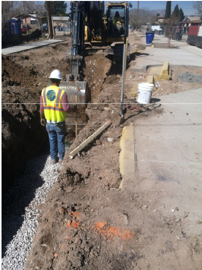
Sanitary Sewer Line Replacement
