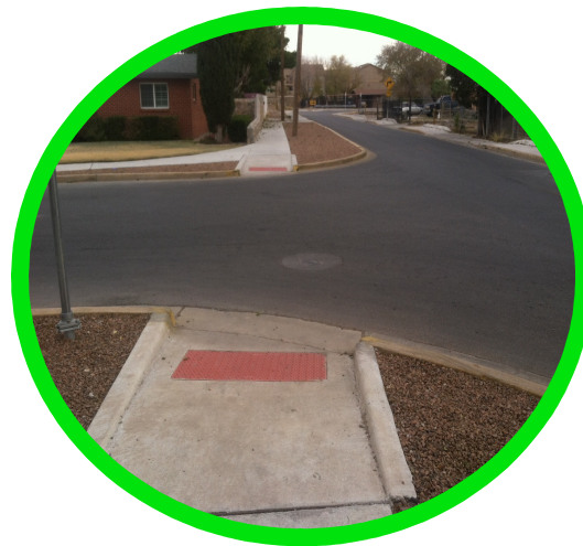
ADA Compliant Directional Curb Ramps
