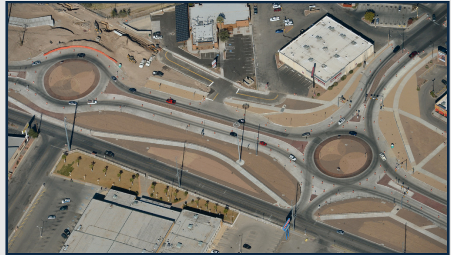
Construction Photos: Lanes open to traffic.
