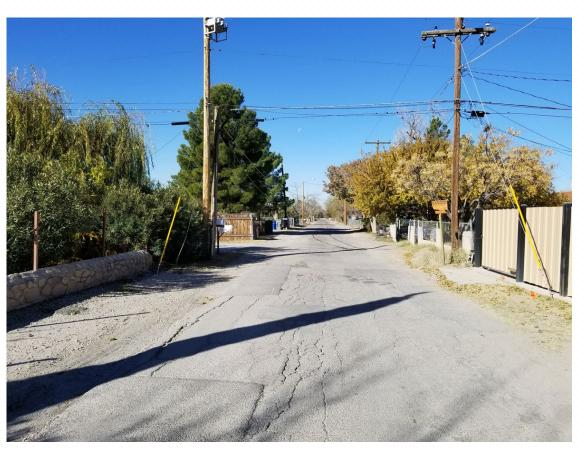
The existing pavement structures exhibit large amount of pavement distress such as rutting, potholes, cracking and segregation.
