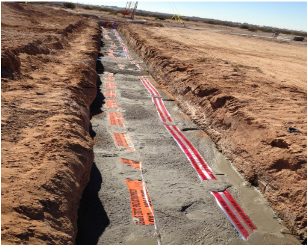
New Airport Surveillance Radar power feeder
