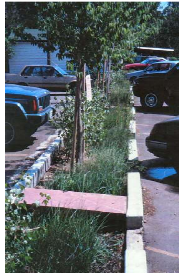
Figure 1-3: This asphalt speed bump redirects stormwater into a vegetated swale. Without the speed bump, stormwater runoff would enter the vegetated swale much lower in the system, bypassing some of the area available for treatment.
