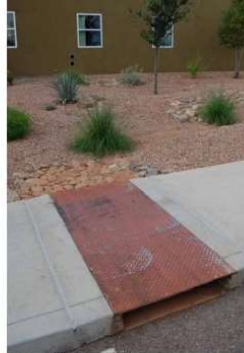
Variations of sidewalk curbs allowing stormwater to flow under sidewalk.
