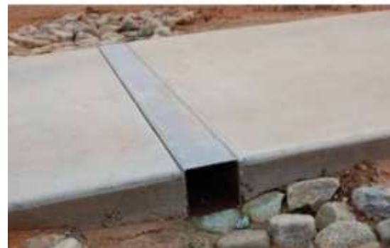
Variations of sidewalk curbs allowing stormwater to flow under sidewalk.
