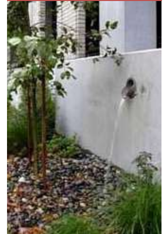
Downspout disconnection
