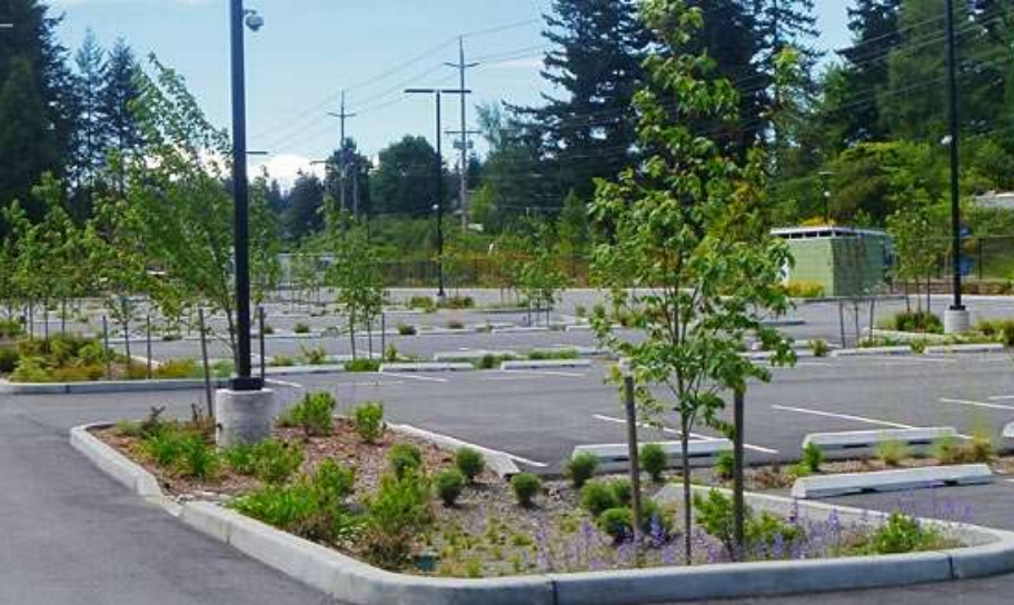
Figure 1-3: This asphalt speed bump redirects stormwater into a vegetated swale. Without the speed bump, stormwater runoff would enter the vegetated swale much lower in the system, bypassing some of the area available for treatment.
