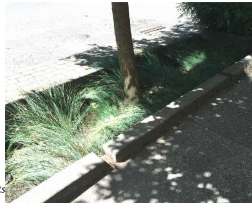
Variations of sidewalk curbs allowing stormwater to flow under sidewalk.
