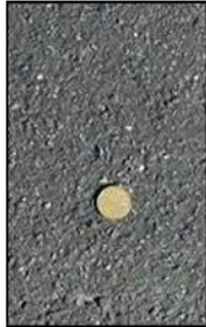
FIGURE B2 Microsurfacing texture one year after construction; diameter of the coin is 1 in.
