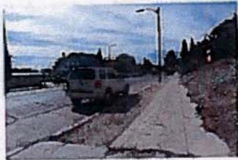
N Montana (Facing West)
