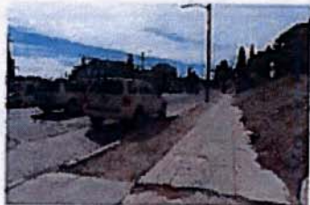
N Montana (Facing West)
