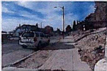
N Montana (Facing West)
