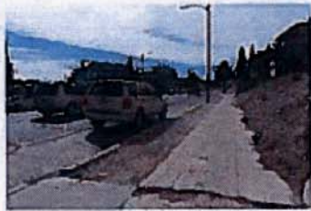
N Montana (Facing West)
