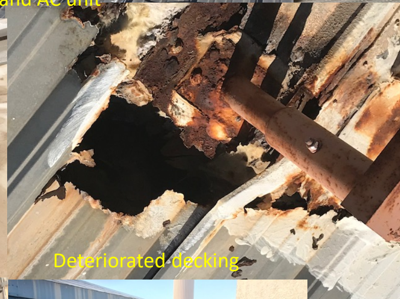
8600 Montana- Deteriorated decking and AC unit
