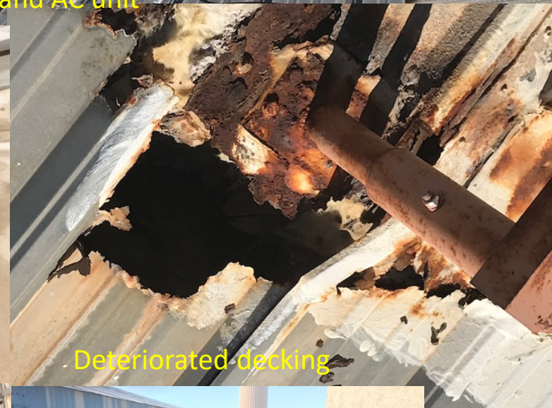
8600 Montana- Deteriorated decking and AC unit
