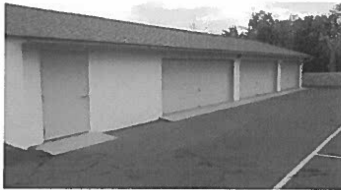
EXISTING FRONT GARAGE ELEVATION PHOTOGRAPH SCALE: NOT TO SCALE
