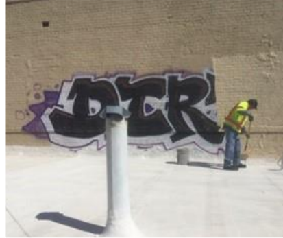
Public Safety Concerns
