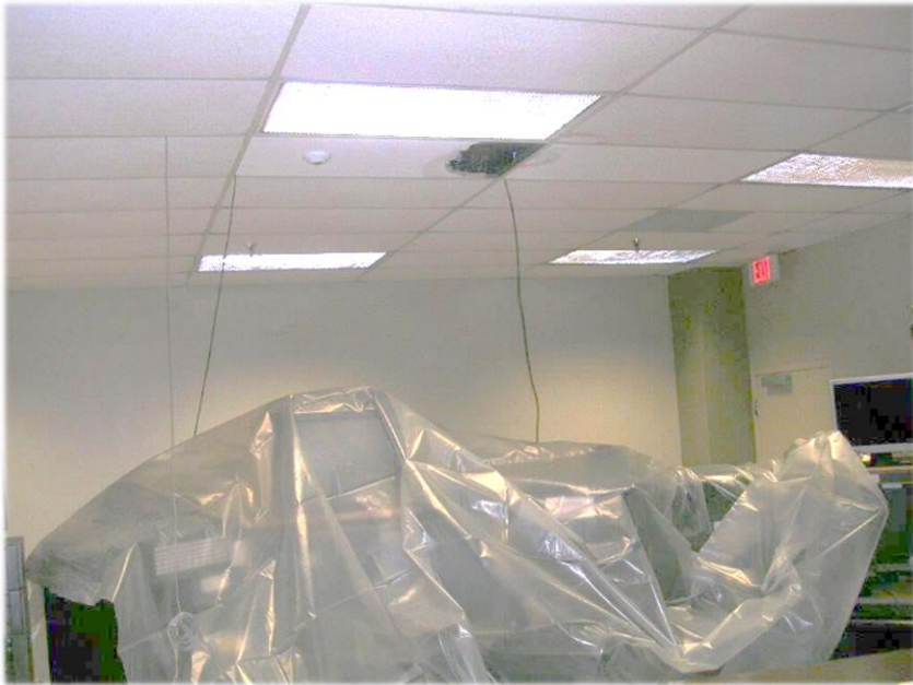
Extensive water damage due to leaking roof
