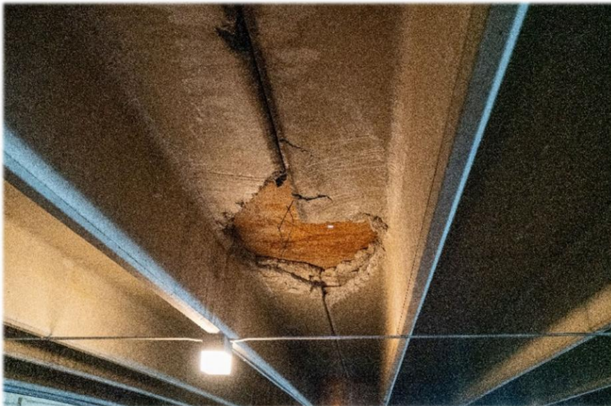
Extensive water damage due to leaking roof
