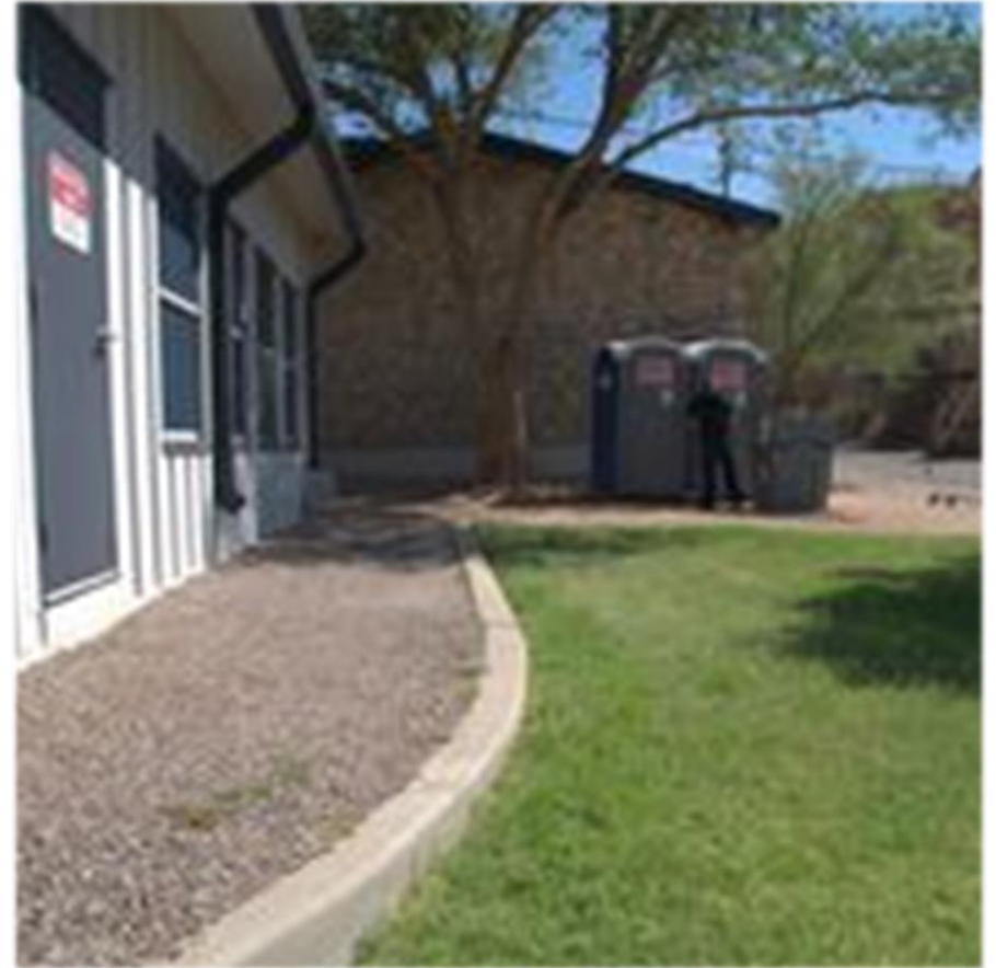
Substandard bathroom facilities
