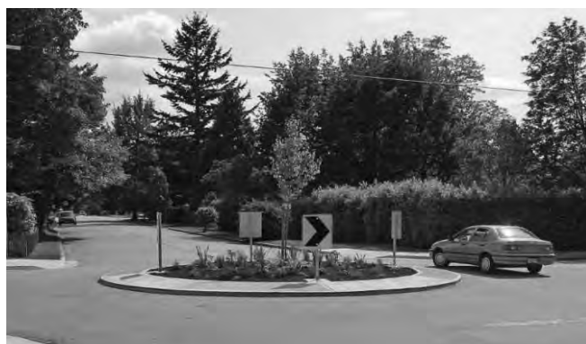
Figure C25. Traffic circles have proven to be effective intersection treatments for bicycle boulevards.
