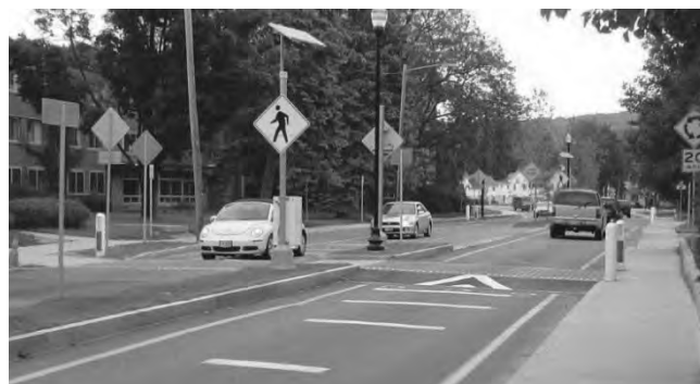
Figure C24. A raised crosswalk doubles as a speed table to reduce motor vehicle speeds.
