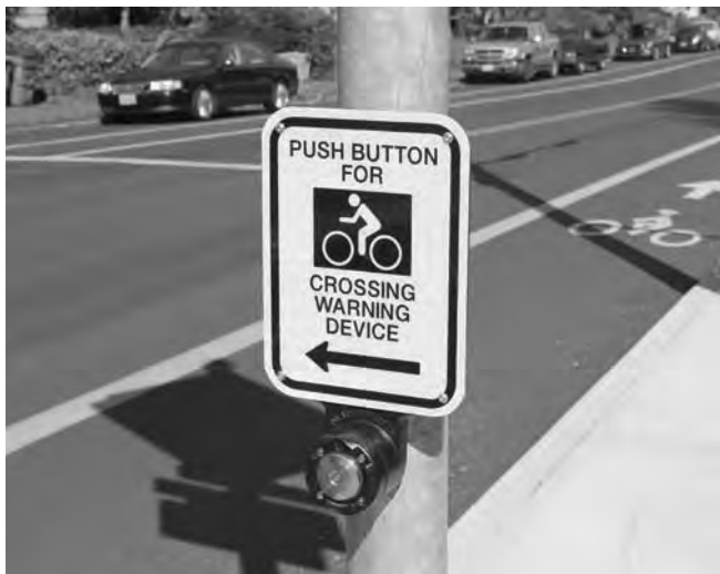
Figure C16. Bicycle push button actuators are positioned to allow bicycle riders in roadway to stop traffic on busy cross-streets.
