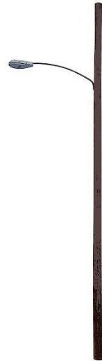
EXISTING LIGHT POLE
