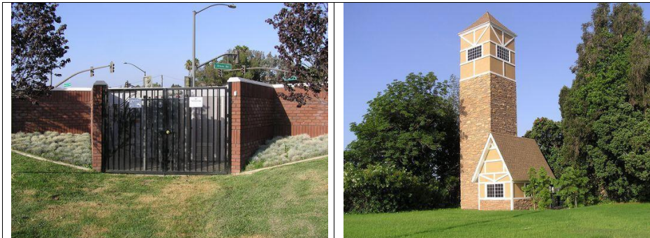
The equipment is move to the edge of the property and screened to blend into the surroundings, as well as another screening example where it is incorporated into the design to blend in.
