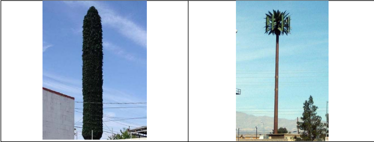
These facilities, while appropriate in the right context, appear to stand out and are not consistent with the scale and development of area.
