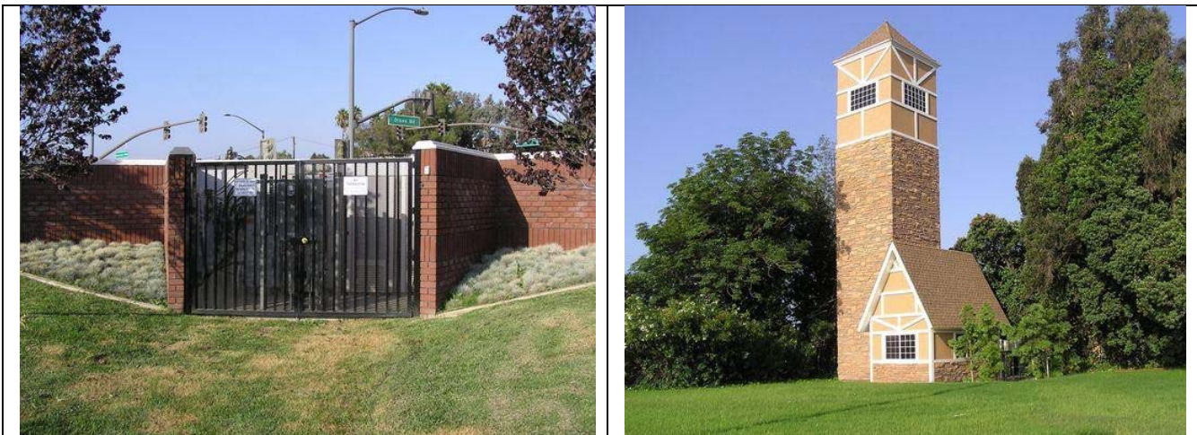
The equipment is move to the edge of the property and screened to blend into the surroundings, as well as another screening example where it is incorporated into the design to blend in.
