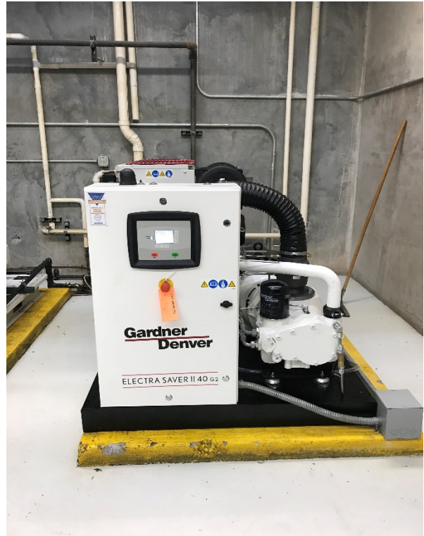
MODEL STG2-40hp ELECTRA SAVER II ROTARY SCREW GENERATION 2 WITH INTENSIVE INJECTION LUBE -460V 3PH 60HZ 125psi - INSTALLED IN 2018.
