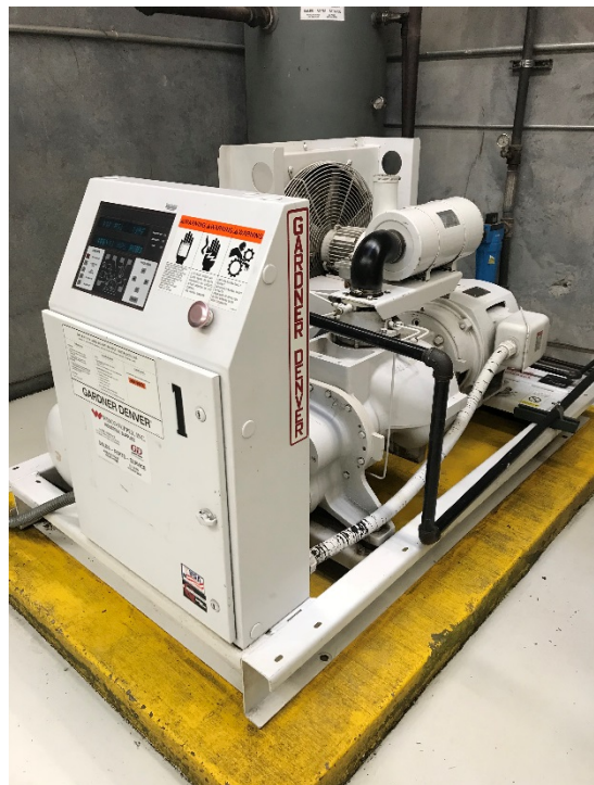
GARDNER DENVER AIR COMPRESSOR UNITS – MODEL ECFQHB AND SERIAL 767663- 1640RPM- 40hp -460V 3PH- 125psi- ROTARY SCREW SINGLE STAGE POSITIVE DISPLACEMENT AIR . INSTALLED IN 2001.
