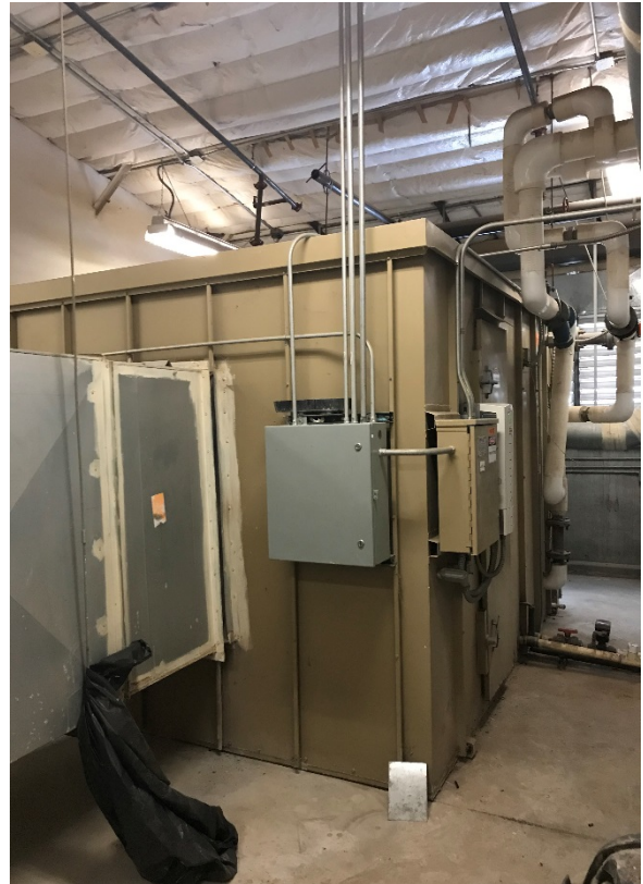
SPEC AIR -AIR WASHER/HEATER UNIT – MODEL #10 460V 3PH 60HZ –LOCATED ON IN THE MAINTENANCE SHOP ON 2ND FLOOR. INSTALLED 2001
