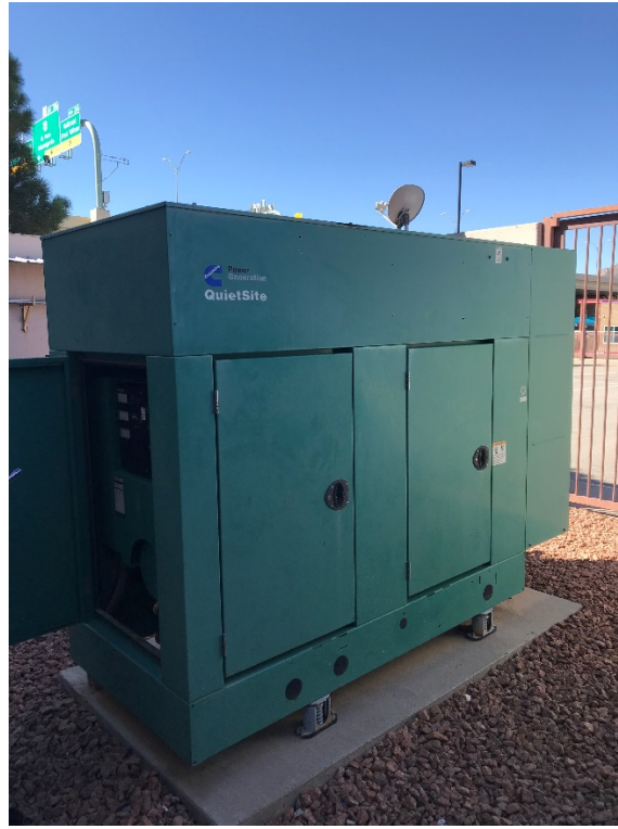
CUMMINS-NATURAL GAS EMERGENCY BACKUP GENERATOR- MODEL GGHE-5003551- 60HZ- 1/3 PHASE RATED- LOCATED WEST SIDE OF THE BUILDING. INSTALLED 2001.
