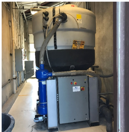
WATER RECOVERY SYSTEM- MODEL DGOELES-CAPACITY 550 GALLONS-ELECTRIC MARATHON MOTOR 230/460V 3PH 60HZ-HIGH PRESSURE CARVER PUMP- INSTALLED IN 2001
