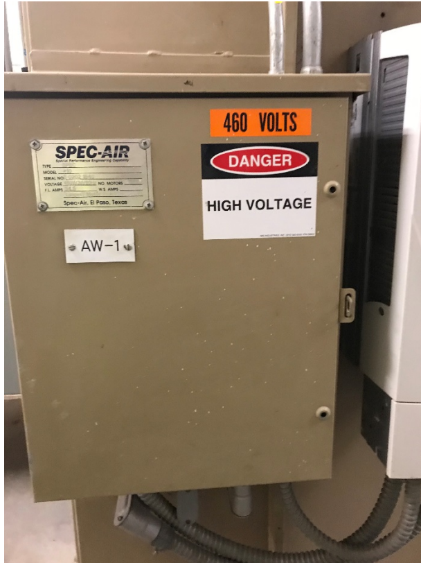
SPEC AIR -AIR WASHER/HEATER UNIT – MODEL #10 460V 3PH 60HZ –LOCATED ON IN THE MAINTENANCE SHOP ON 2ND FLOOR. INSTALLED 2001
