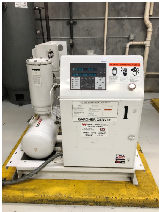
GARDNER DENVER AIR COMPRESSOR UNITS – MODEL ECFQHB AND SERIAL 767663- 1640RPM- 40hp -460V 3PH- 125psi- ROTARY SCREW SINGLE STAGE POSITIVE DISPLACEMENT AIR . INSTALLED IN 2001.
