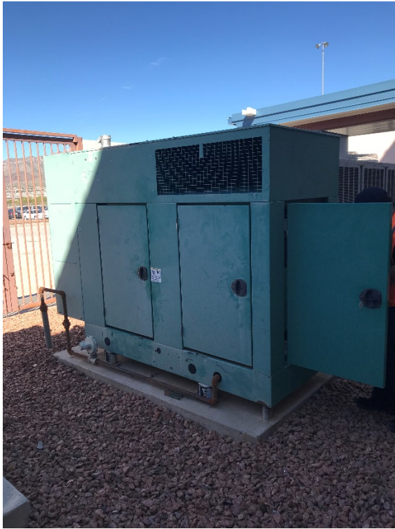
CUMMINS-NATURAL GAS EMERGENCY BACKUP GENERATOR- MODEL GGHE-5003551- 60HZ- 1/3 PHASE RATED- LOCATED WEST SIDE OF THE BUILDING. INSTALLED 2001.
