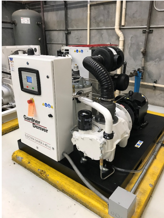
MODEL STG2-40hp ELECTRA SAVER II ROTARY SCREW GENERATION 2 WITH INTENSIVE INJECTION LUBE -460V 3PH 60HZ 125psi - INSTALLED IN 2018.
