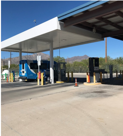
TWO ANGI CNG DISPENSERS –TWO CT-1000 CNG NOZZLES INSTALLED PER DISPENSER ( TOTAL OF 4 CNG NOZZLES)– WHITE TULSA CNG DISPENSER IS NOT OPERABLE-PART OF DECOMMISSIONED LCNG STATION. ANGI DISPENSERS INSTALLED IN 2013.
