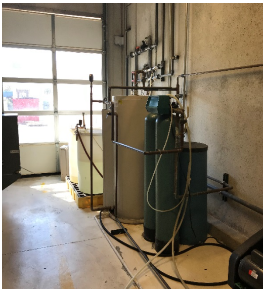
WATER RECOVERY SYSTEM- MODEL DGOELES-CAPACITY 550 GALLONS-ELECTRIC MARATHON MOTOR 230/460V 3PH 60HZ-HIGH PRESSURE CARVER PUMP- INSTALLED IN 2001
