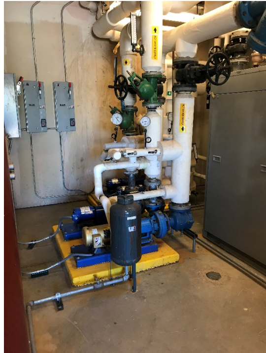
THESE RECIRCULATION PUMPS ARE PART OF THE BRYAN BOILER UNIT UP ABOVE- TWO US ELECTRIC 2 h.p. 230/460V MOTORS- FRAME 145T AND TWO STERLING WATER PUMPS MODEL F1825 6.75in. LOCATED IN MECHANICAL ROOM ON NORTH SIDE OF THE BUILDING. INSTALLED IN 2001.
