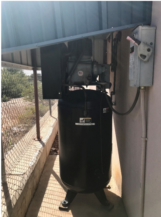
GARDNER DENVER MODEL M3311T-CH 80 gal AIR COMPRESSOR –MAWP 200psi-230/460V 1PH 60HZ BALDOR MOTOR 7.5 hp-LOCATED EAST SIDE OF THE SERVICE/STORAGE AREA. INSTALLED IN 2001
