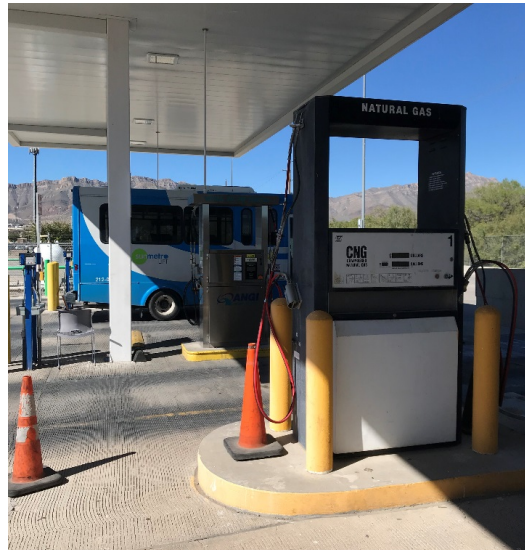
TWO ANGI CNG DISPENSERS –TWO CT-1000 CNG NOZZLES INSTALLED PER DISPENSER ( TOTAL OF 4 CNG NOZZLES)– WHITE TULSA CNG DISPENSER IS NOT OPERABLE-PART OF DECOMMISSIONED LCNG STATION. ANGI DISPENSERS INSTALLED IN 2013.
