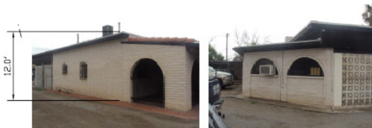
MAIN BUILDING - SIDE VIEW
