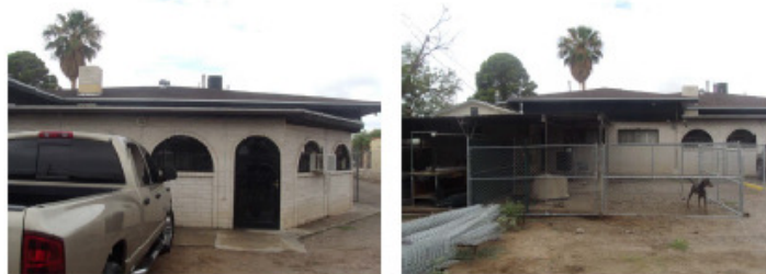
MAIN BUILDING - BACK VIEW
