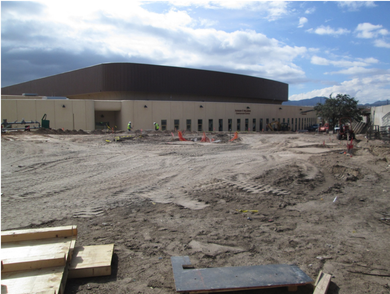
Underground conduits complete, final grading to follow
