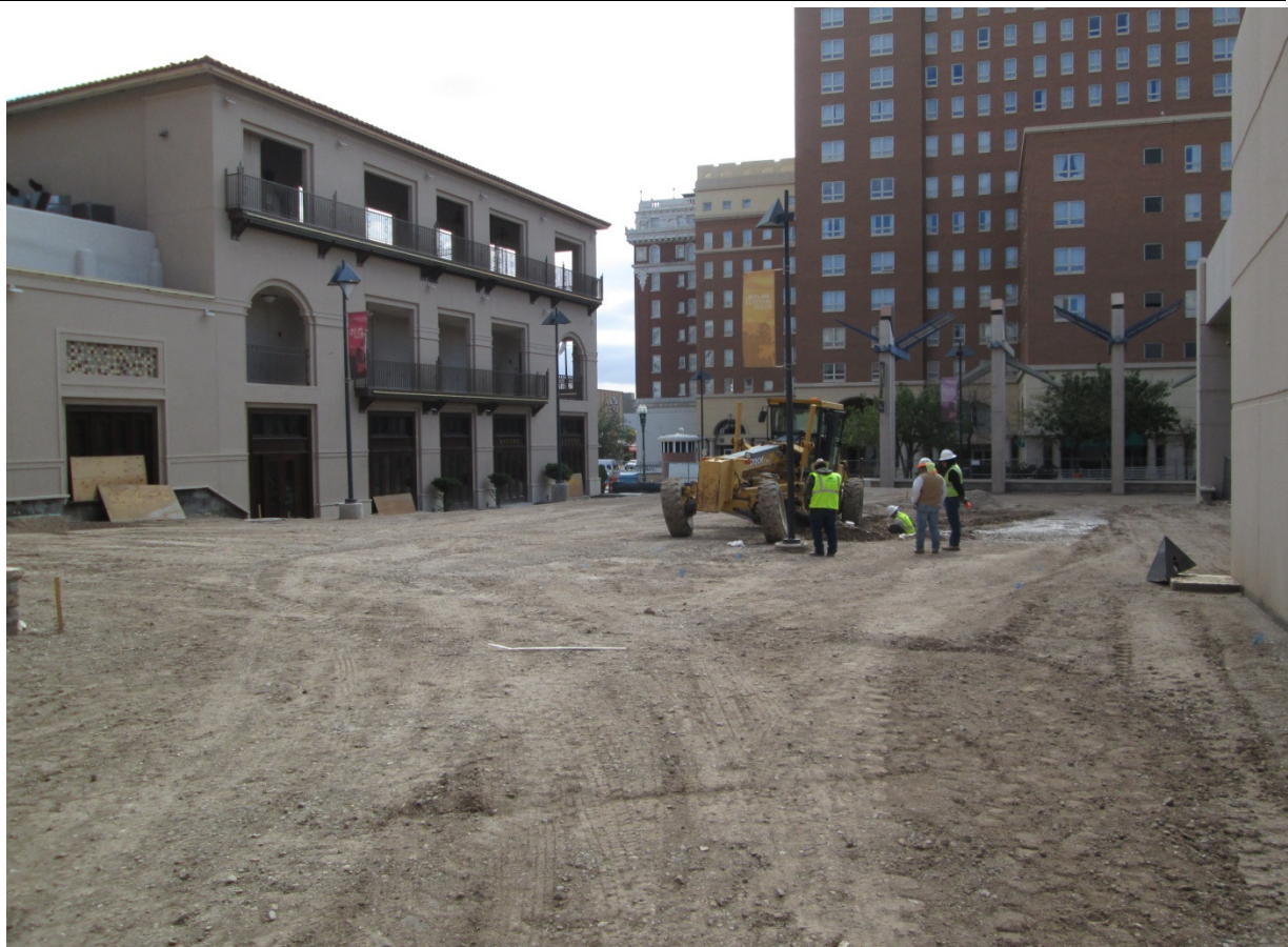
Rough grading complete, underground conduits to follow
