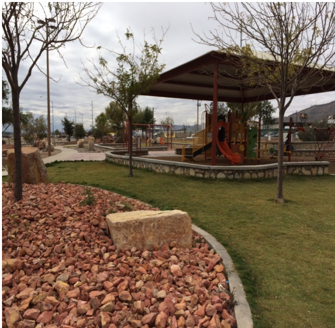
New playground equipment and new metal shade canopy installation
