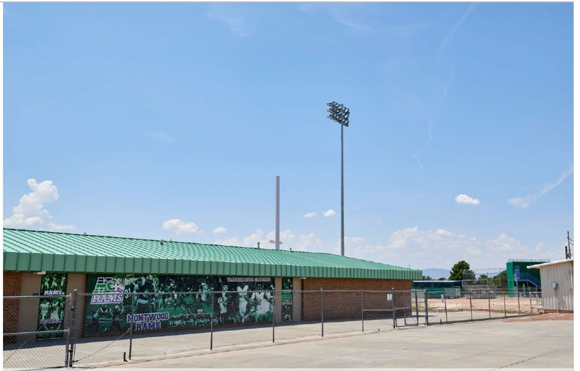
PHOTO SIMULATION NOT TO SCALE. ALL DIMENSIONS ARE APPROXIMATE BASED ON 3D IMAGING AND KNOWN HEIGHT OF ADJACENT STRUCTURE.
