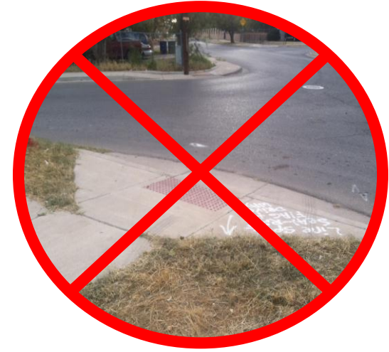
Diagonal Curb Ramps No Longer Desired
