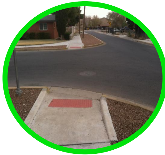
ADA Compliant Directional Curb Ramps
