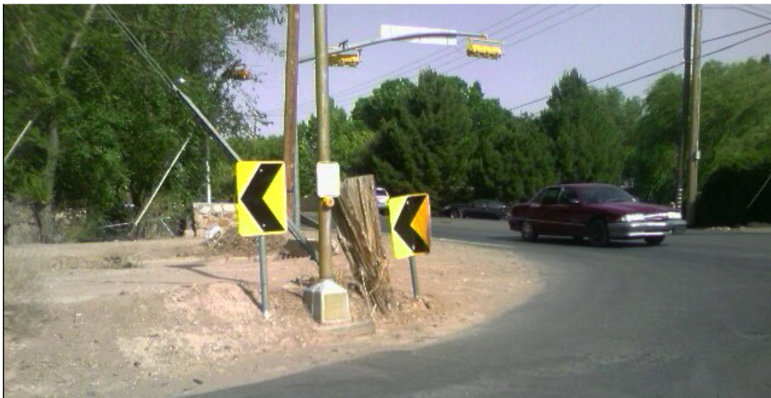
Figure 12: Inaccessible Pedestrian Push Button at Country Club and Montoya
