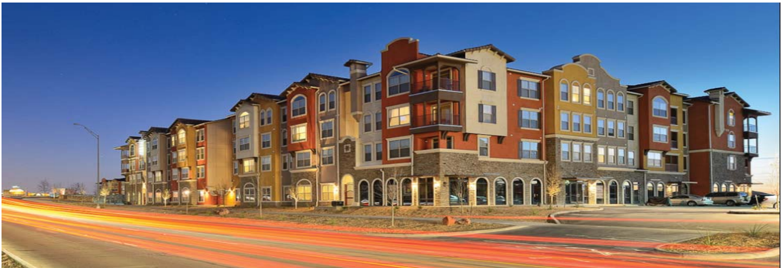
The Venue at Montecillo, El Paso
